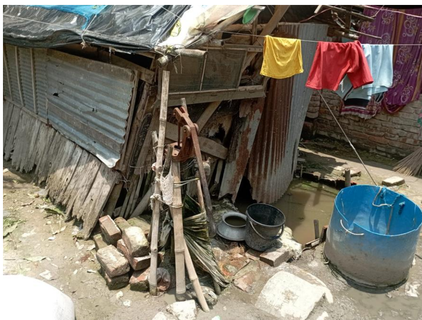
A fragile, makeshift setup in Satkhira where a tube well—intended to provide safe drinking water—is precariously supported with bamboo poles, bricks, and string. Ashashuni, Satkhira, May 2025. © Amnesty International
