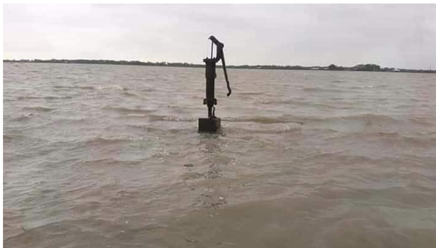
A tubewell completely submerged in flood water. Floods render tubewells unusable for weeks, pushing already-excluded Dalit communities to unsafe alternatives like pond water or contaminated shallow wells. The image reflects how climate change intensifies water insecurity in these vulnerable regions. Photo: Paritran. Khulna © Amnesty International
