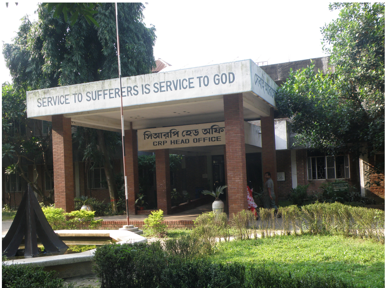
Rehabilitation Center for victims of Rana Placa Collapse in Savar (2013).
